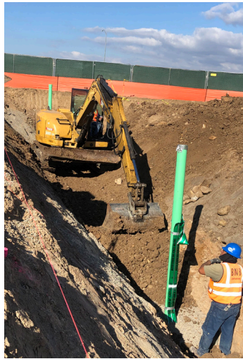
Trenches being dug in preparation for new Automotive Technology Program facilities.
