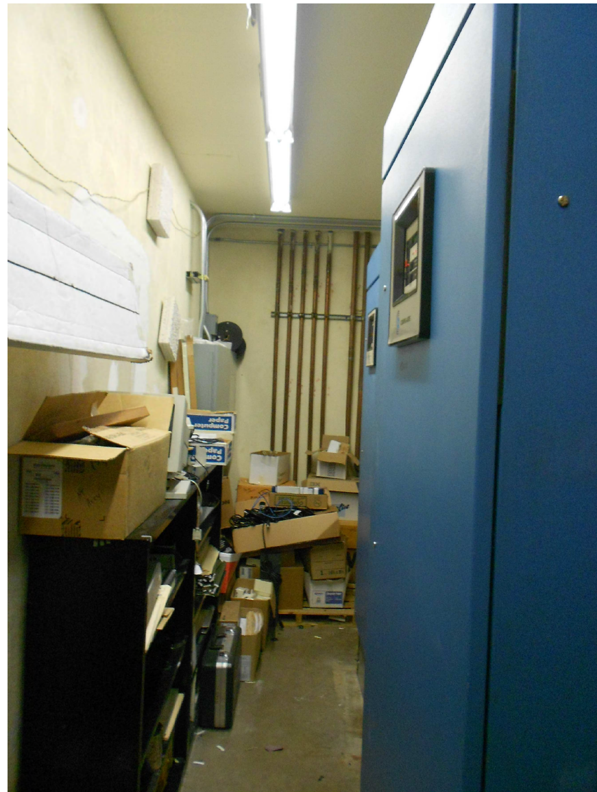
EXISTING CRAC UNIT TO BE REMOVED 13
