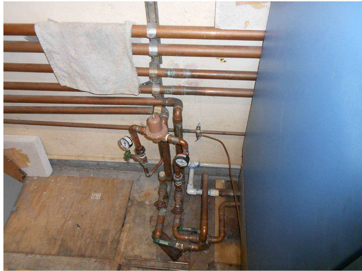
REFRIGERANT PIPING CONNECTED TO CRAC UNIT TO BE REMOVED 6
