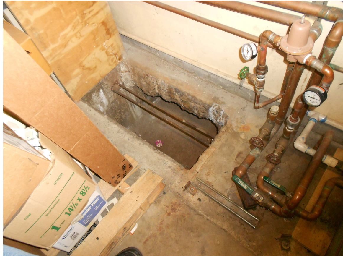
OPENING IN FLOOR SLAB OF RM-211L 7
