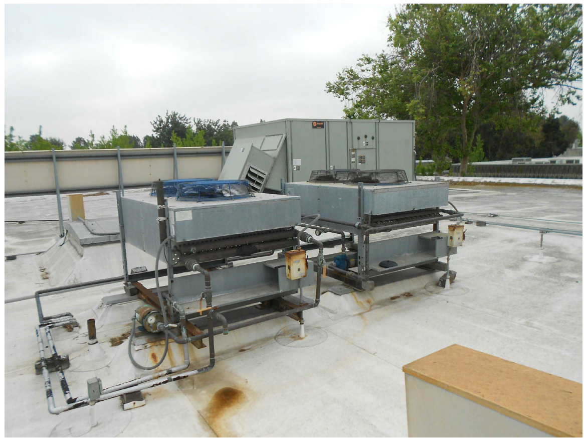
CONDENSING UNITS ON ROOF TO BE REMOVED 4
