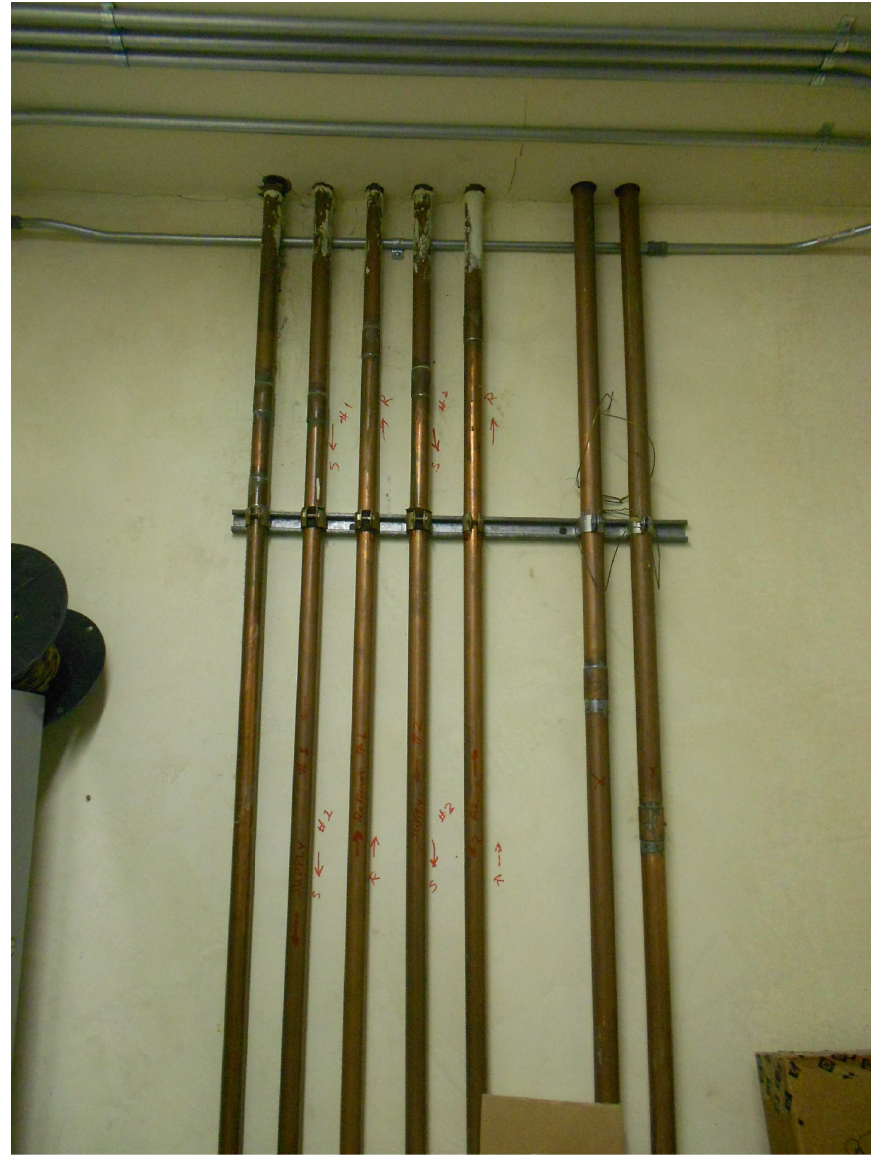
REFRIGERANT PIPING TO CONDENSING UNIT ON ROOF TO BE REMOVED 12
