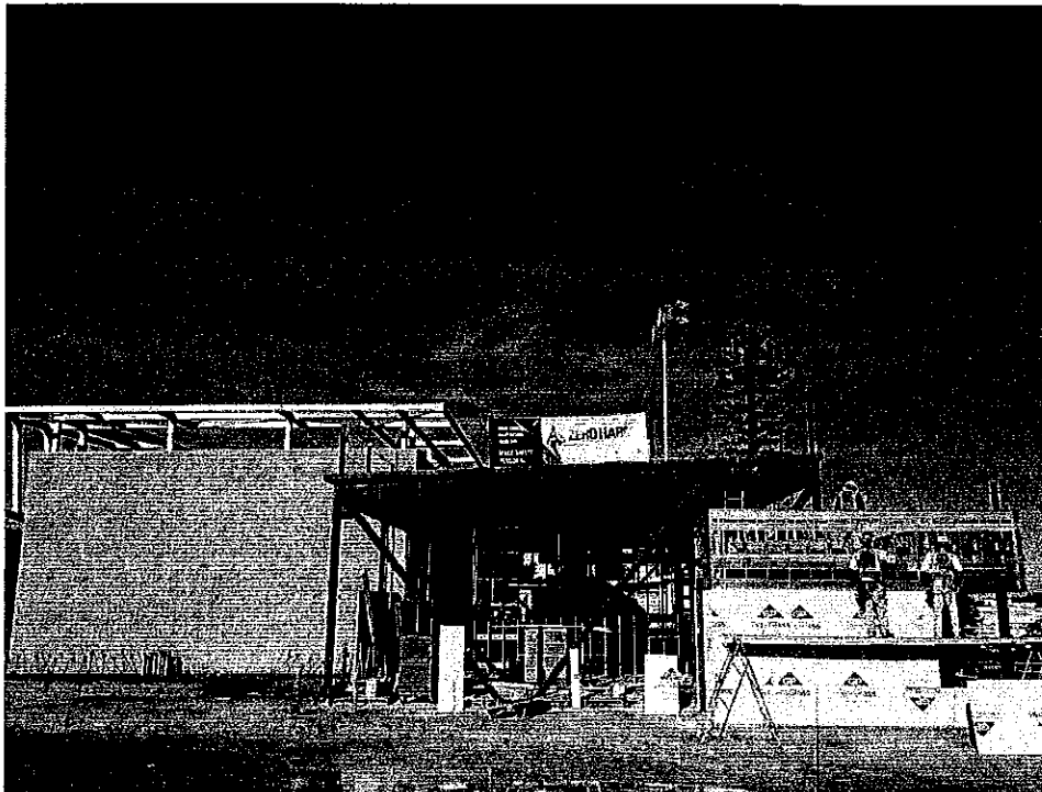
DensGlass wall exterior sub-framing looking at corner of ticket booth area
