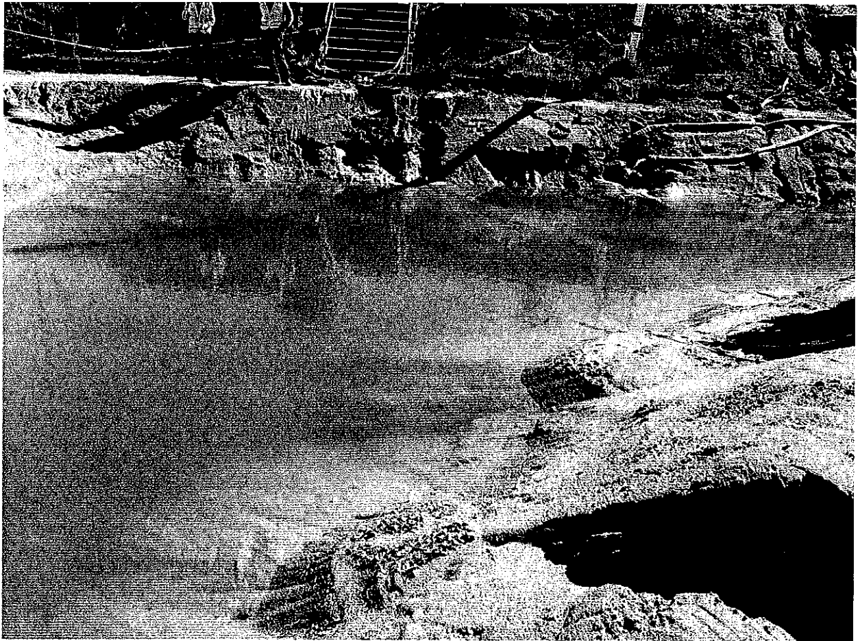
Temporary water basin pond for dewatering effort
